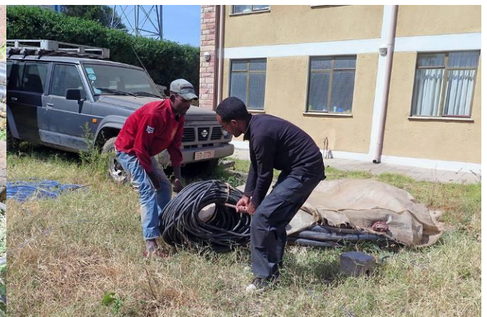
handling the cable
