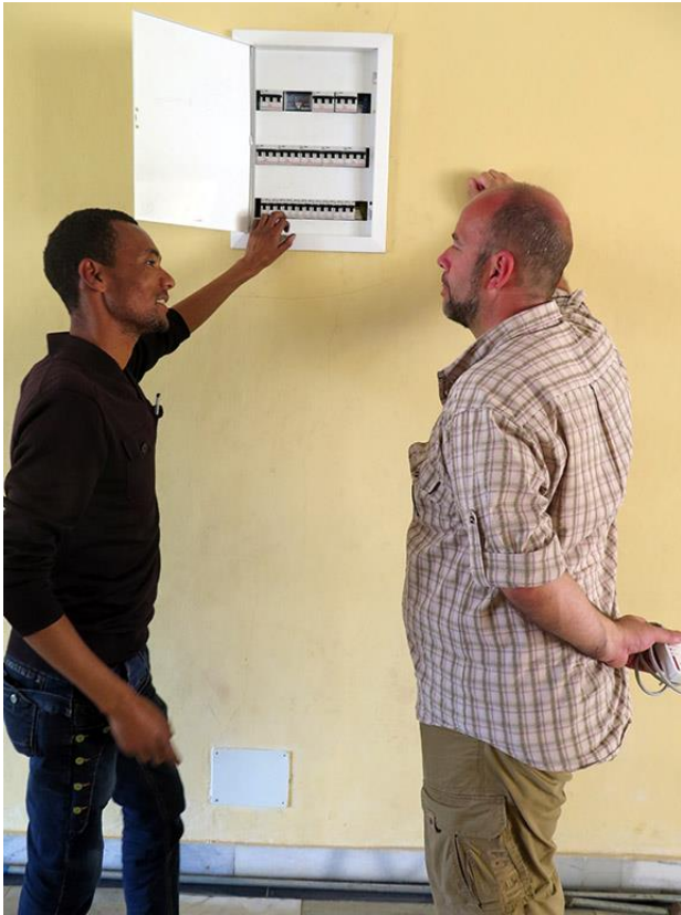
clarification with an electrician
