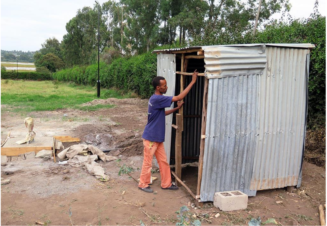
Control house nearly finished
