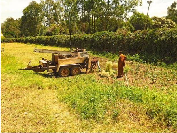
start preparing the ground
