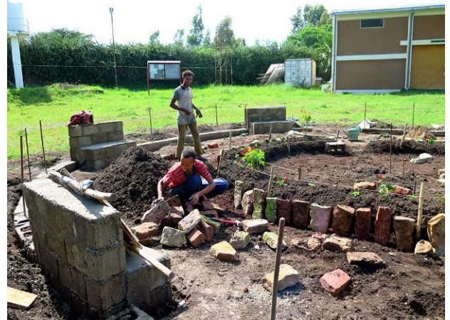
beginning of the works
